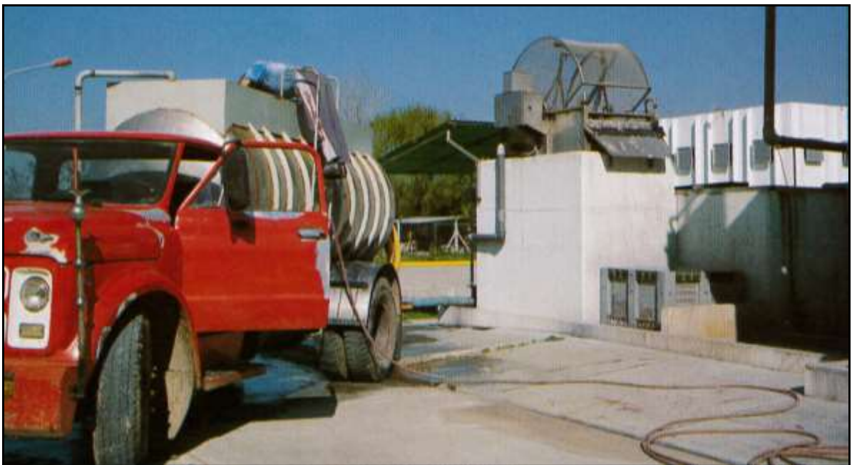
Chrome recovery plant during the activities
