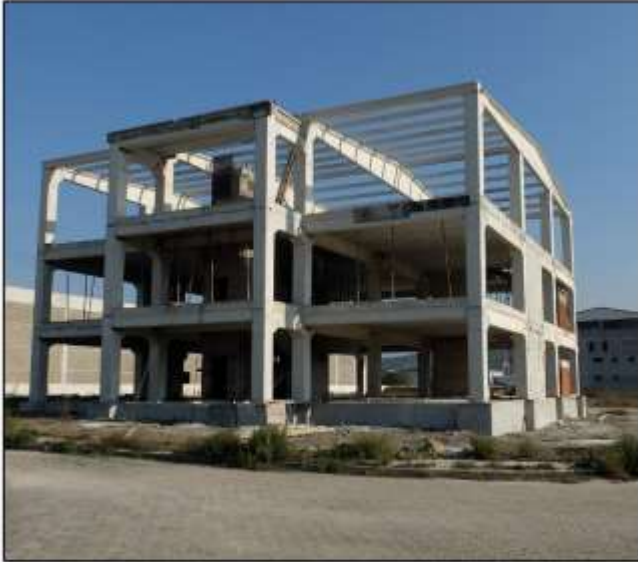
Tannery under construction
