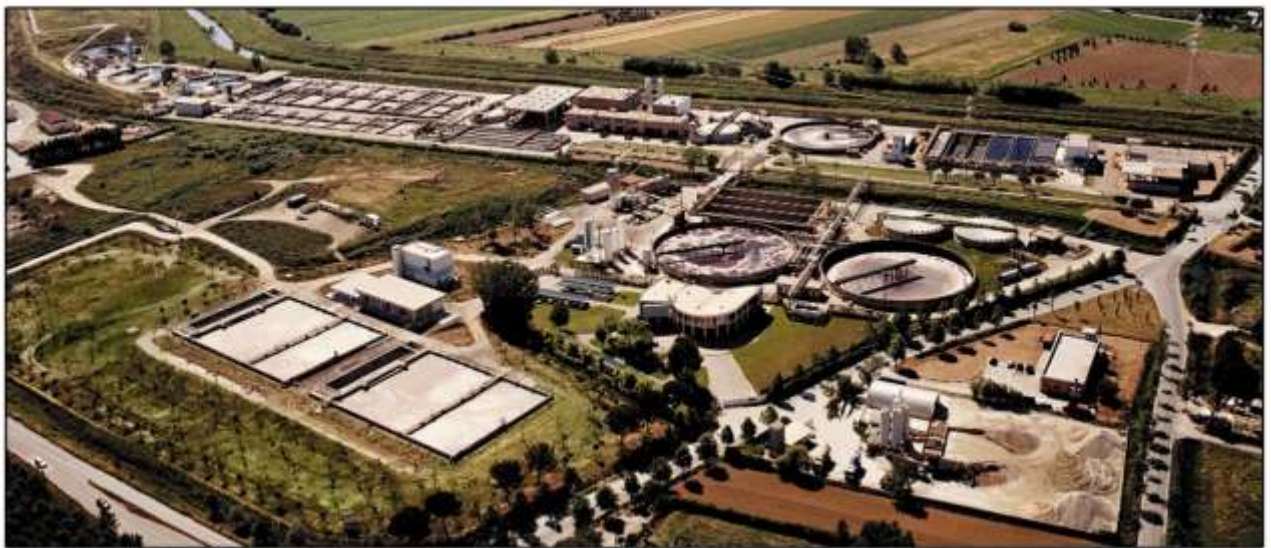
Aquarno CETP - Aerial view
