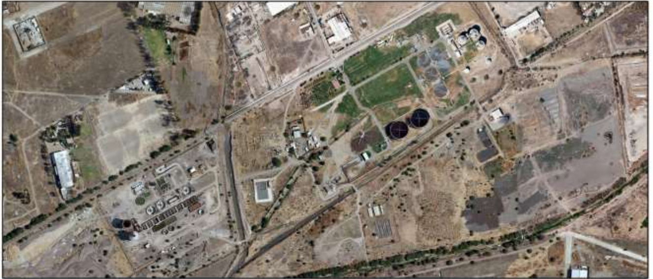
Satellite view of the central effluent treatment plant
