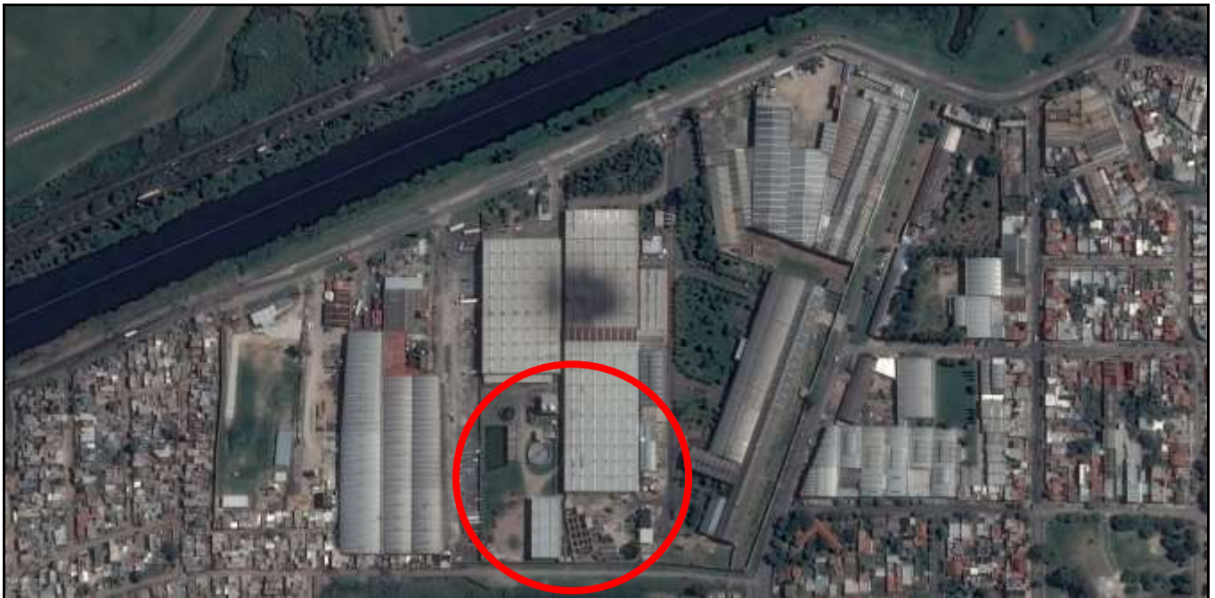
Private individual treatment plant recently built
