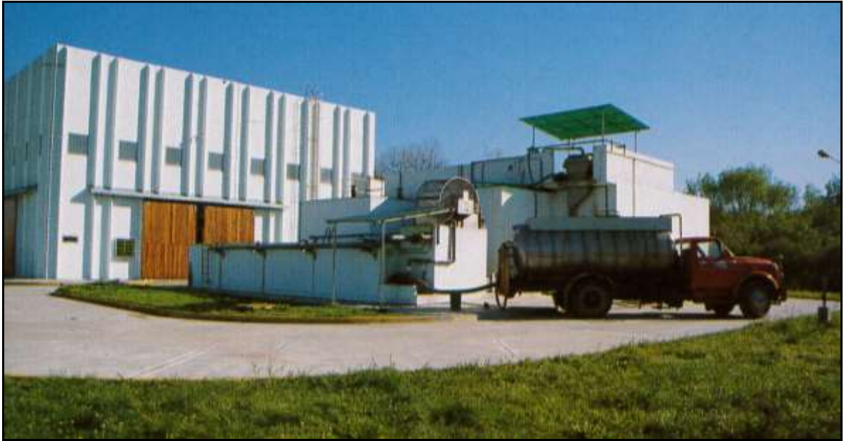
Chrome recovery plant during the activities
