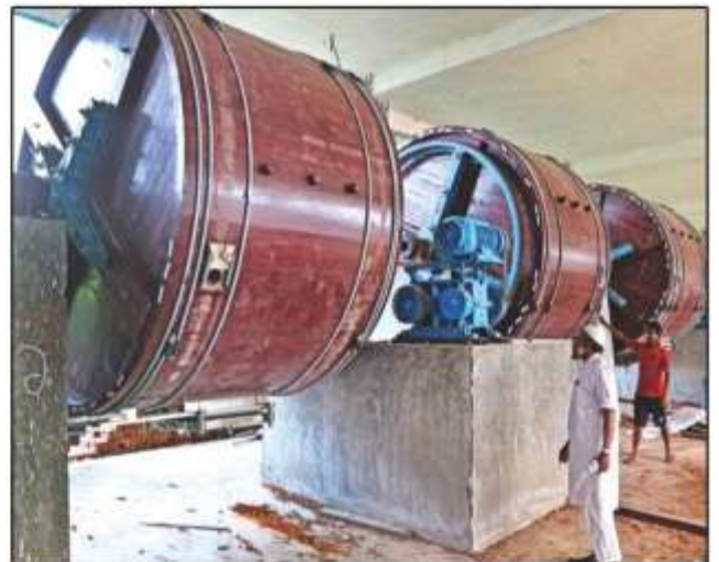
Drums installation - work in progress
