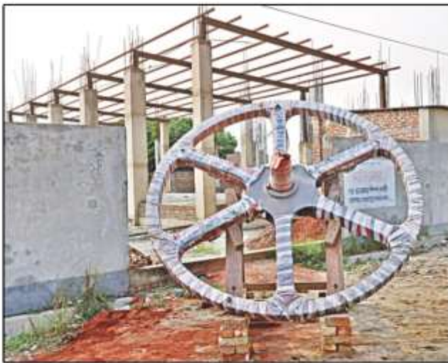
Drums installation - work in progress
