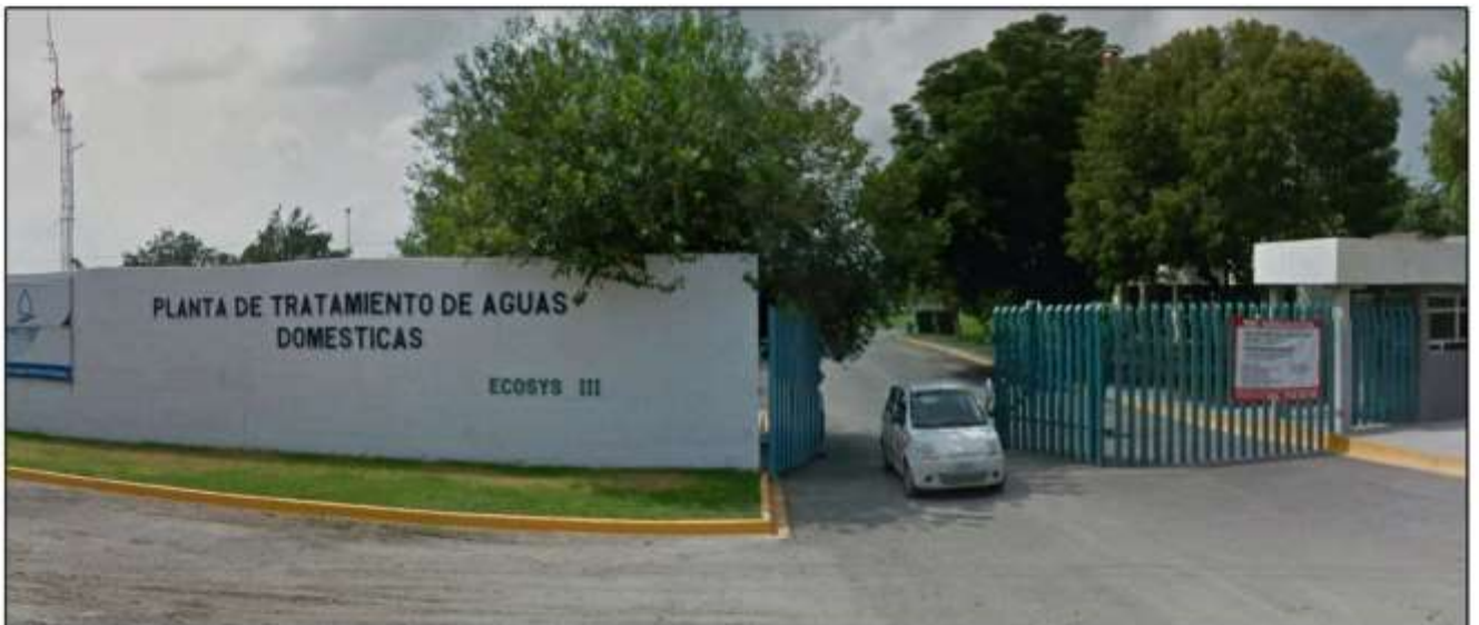
Central effluent treatment plant access
