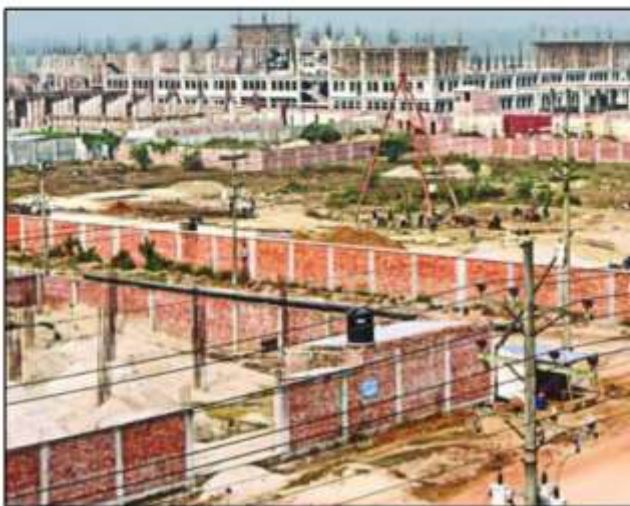
Tanneries under construction in Savar
