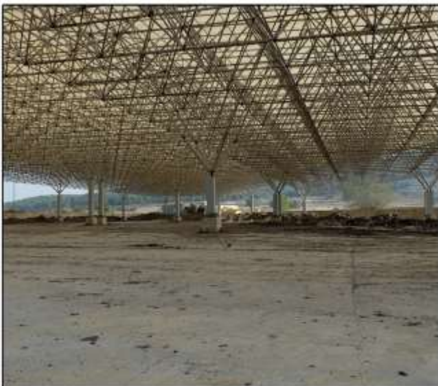
Bursa landfill with CETP sludge store
