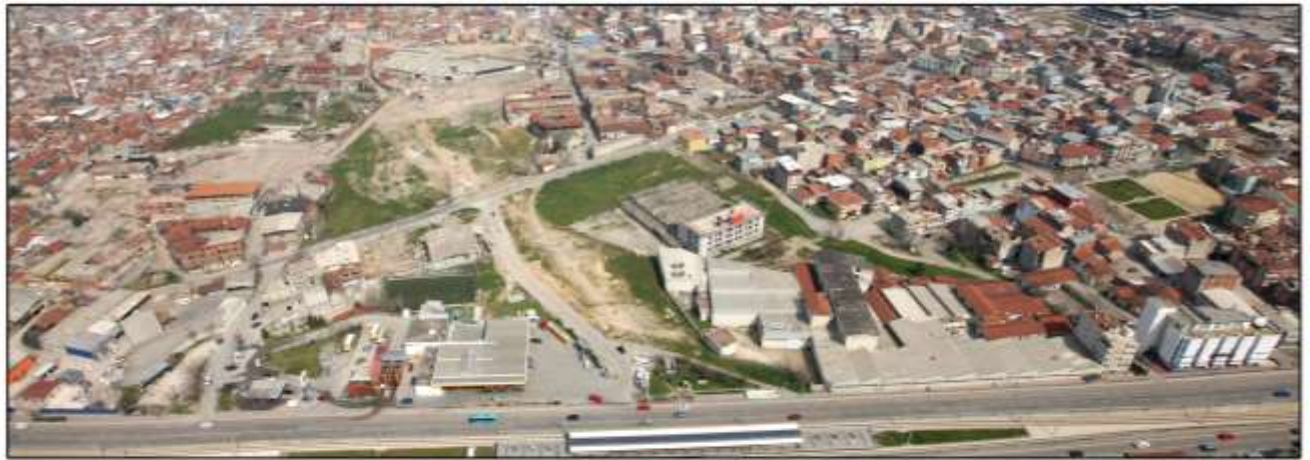
Bursa old tannery are - aerial view
