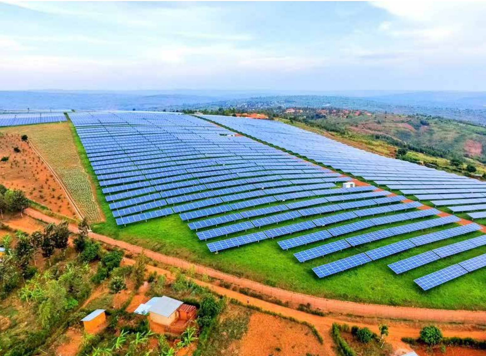
© Solar Plant Rwamagana. Photo by Vifo Rwanda Ltd
